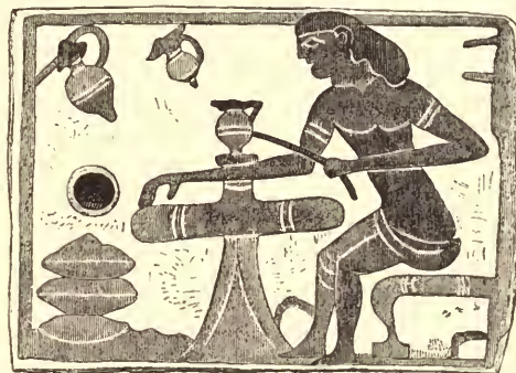
FIG. 20.—Votive tablet from Corinth, full size; a potter applying painted bands while the vessel revolves on the wheel.
