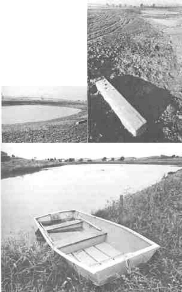
streams may be inundated in flood times, and often have gravelly bottoms that will not hold water very well. But banks can be built up to exclude floodwater, and as long as water flows from the creek into the pond through the inlet pipe, inflow can usually be regulated to balance seepage.)
