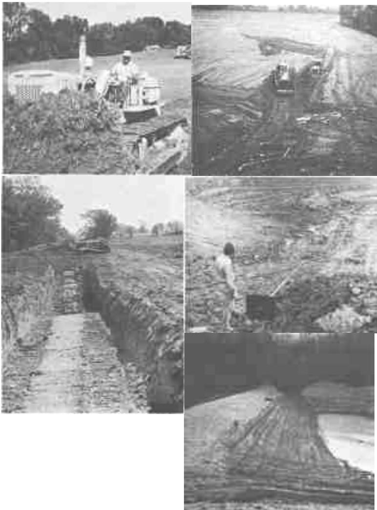
*Construction of an embankment pond involves heavy earth-moving equipment. The first step is to clear the pond area of vegetation and strip the topsoil. Then the core trench is excavated, to be filled, as the embankment is heaped up, with impervious clay. Any pipes passing through the core of the dam are placed and fitted with antiseep collars. Eventually the embankment grading is completed, and the pond starts to accumulate water.*
