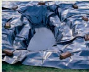
**1** Dig a shallow hole with a sloping edge and shelved sections for access and gradients. Line the hole with a pond liner and temporarily weigh it down.
