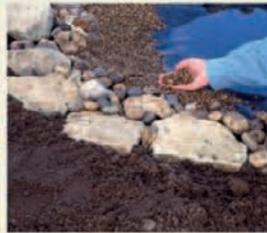
**2** Cover the liner with sand, soil, and gravel. Ideally, fill the pond with rainwater from water butts, or allow it to fill naturally with rain.
