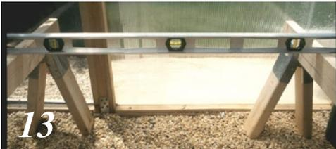
**Step13.** Assemble your stand from 2 saw horse kits and some 2x4 lumber. Use a level placed between the two saw horses to make sure the chambers will lay flat, with zero slope.
