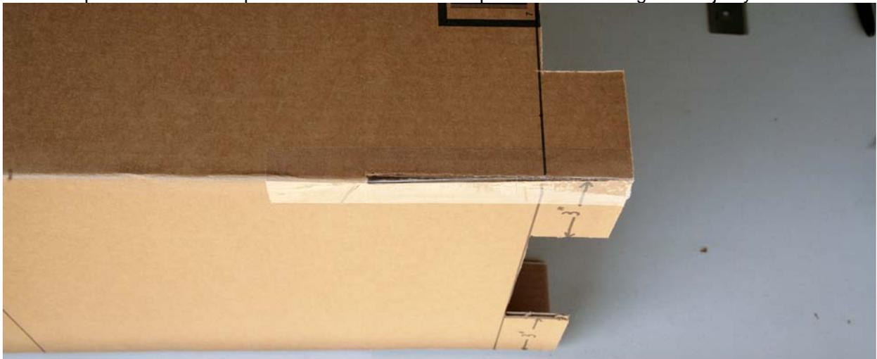
6. After all 4 corners have been taped along the vertical corners of the box, cut a 9" or 10" length of 2" wide tape and wrap it around the 3" corners trying to maintain about the same amount of excess tape on each end as shown below.
