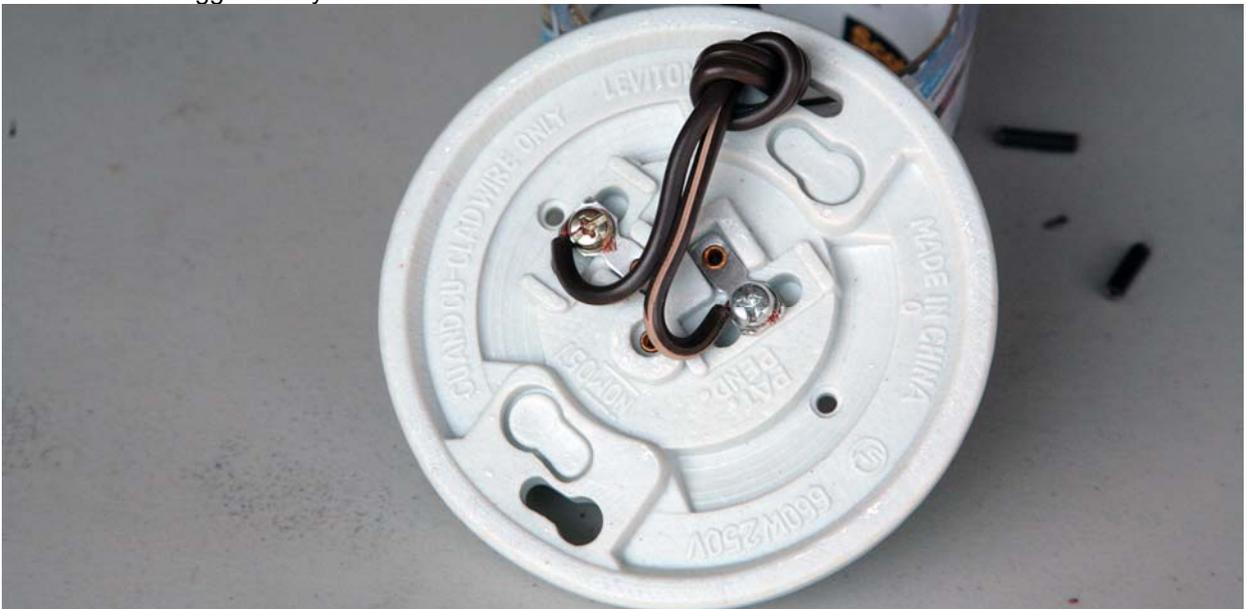
9. Mount the lamp holder to the pancake electrical box using the long 8-32 screws supplied with the lamp holder. Make sure that the knot you tied in the electrical cord is inside the box and not pinched between the edge of the box and the lamp holder. Make sure the screws are snug but do not over tighten as this could crack the lamp holder.
